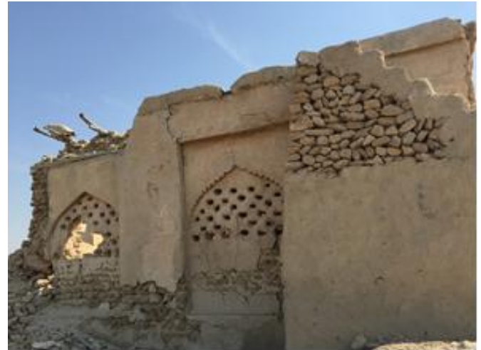
Figure 38. Using coquina in diagonal line, Bassidu village, Qeshm Island (Photographed by Zohreh Moradi).
