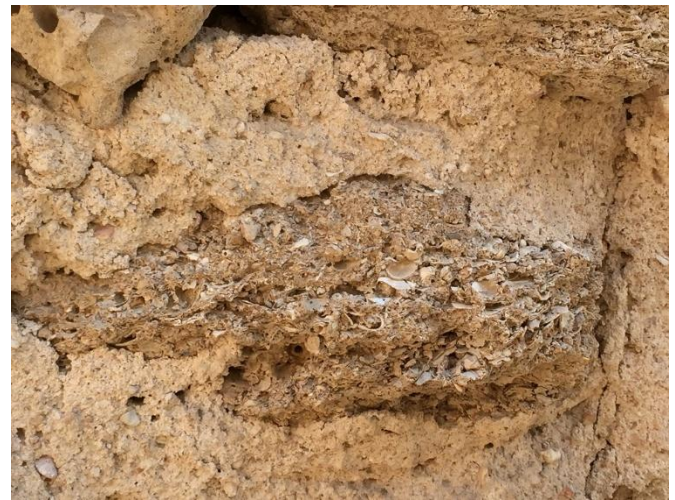
Figure 39. Coral and shells in coquina, Basaidu, village Qeshm Island (Photographed by Zohreh Moradi).
